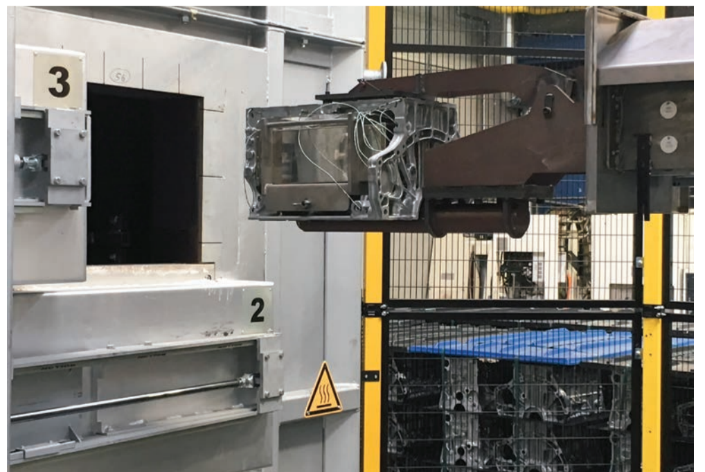
Component and PhoenixTM system being loaded into furnace by gripper
